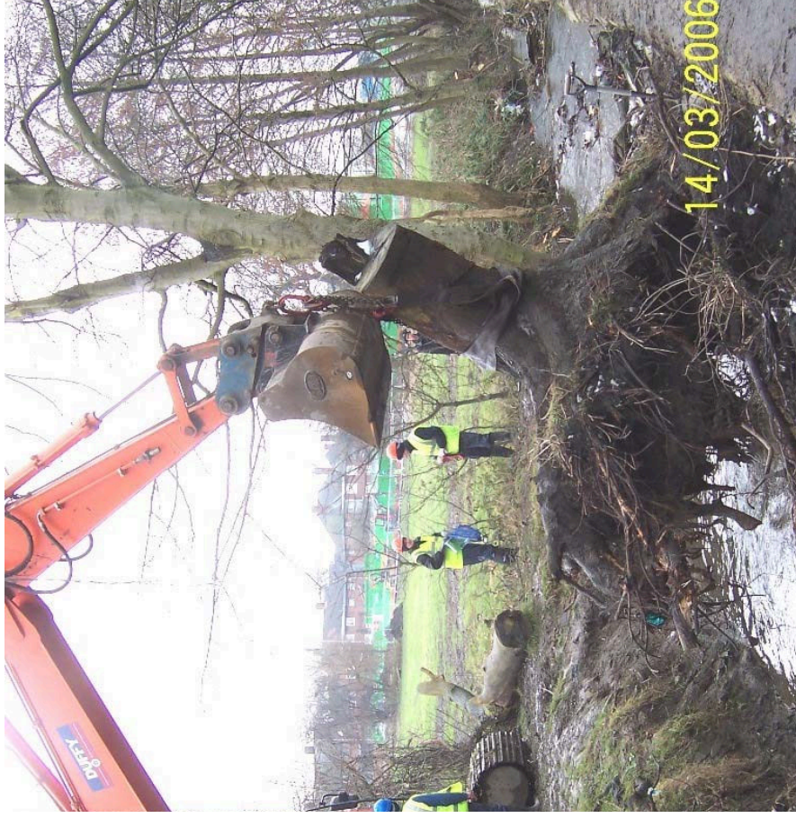
Removal of a mature tree from the centre of Wyke Beck (behind the Foxwoods) as part of the planned maintenance. Flooding in May 2005 affected properties adjacent to this stretch of beck
